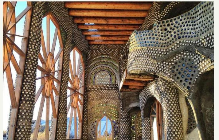
A wide range of materials can be used in the construction of this center, such as: glass bottles, car tires, aluminum cans, wooden pallets, hemp blocks, recycled plastic blocks and beams, ecological bricks made from recycled cardboard and cement, straw bales, and adobe, among others.
